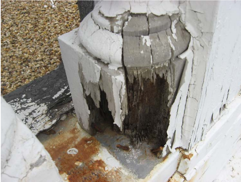
Photo P17-1 – Severely deteriorated wood baluster.
