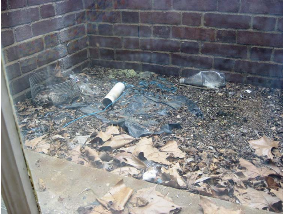
Photo P15-1 – Debris at areaway, south side of building.
