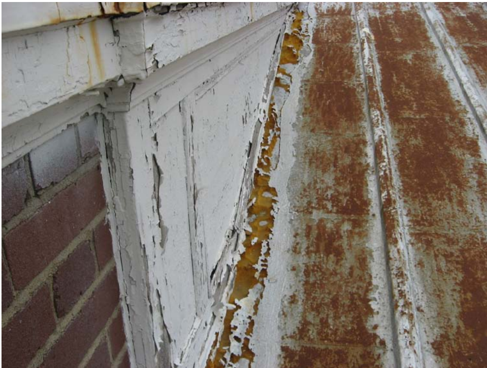
Photo P16-2 – Deteriorated flashing at portico roof-to-parapet wall connection.
