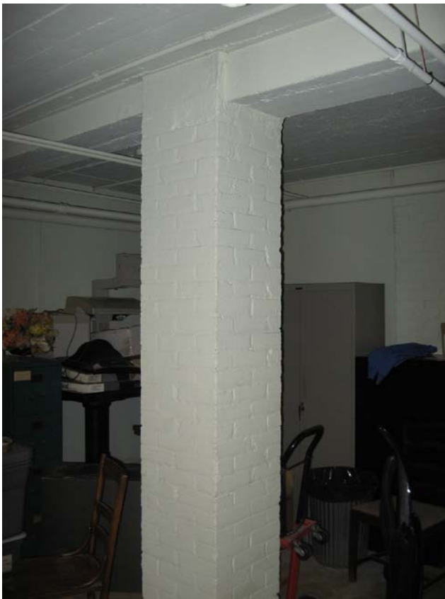
Photo P3-2 – Typical masonry columns at Basement.
