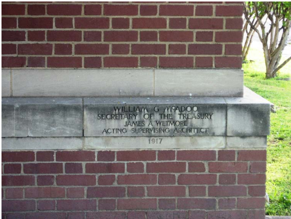
Photo P1-2 – Limestone water table at First Floor Level.
