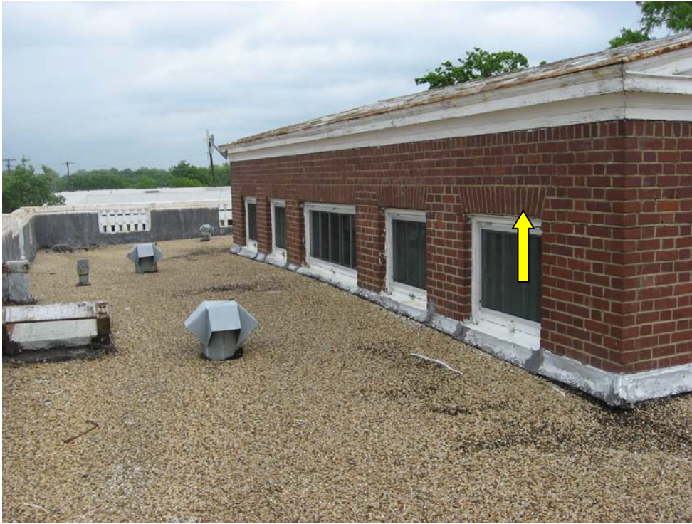
P9-1 – Deteriorated brick mortar joints, West Elevation, Second Floor.
