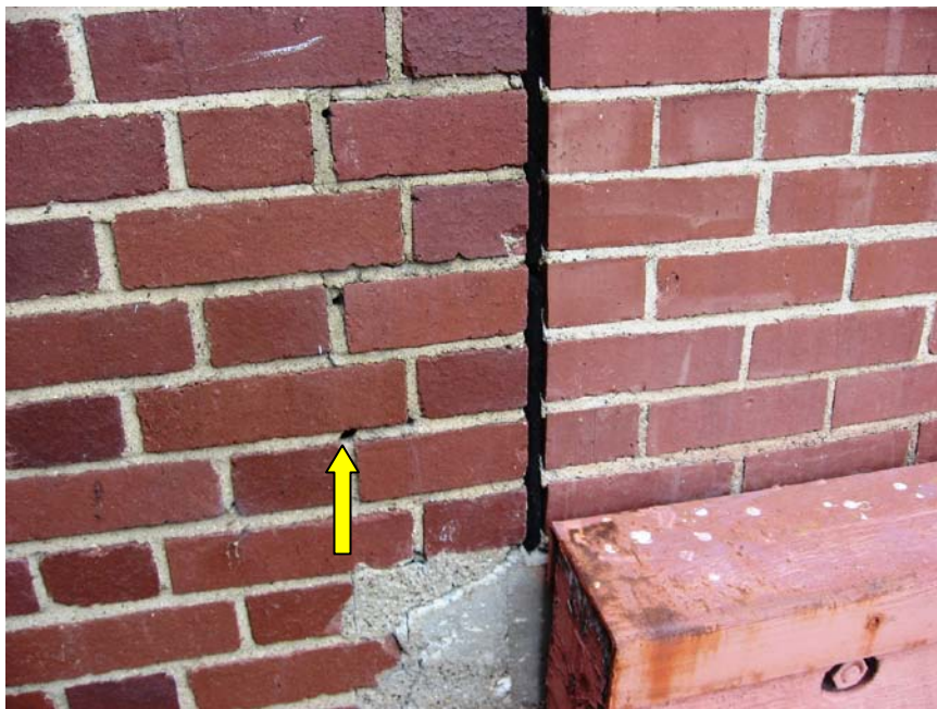
Photo P10-2 – Minor holes in mortar joints, South Elevation. Note joint is not adequately sealed.
