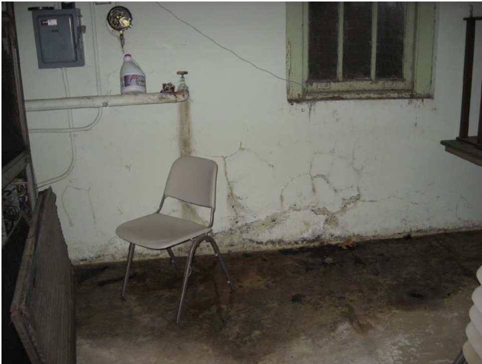
Photo P20-2 – Water infiltration along west wall, Basement Level.
