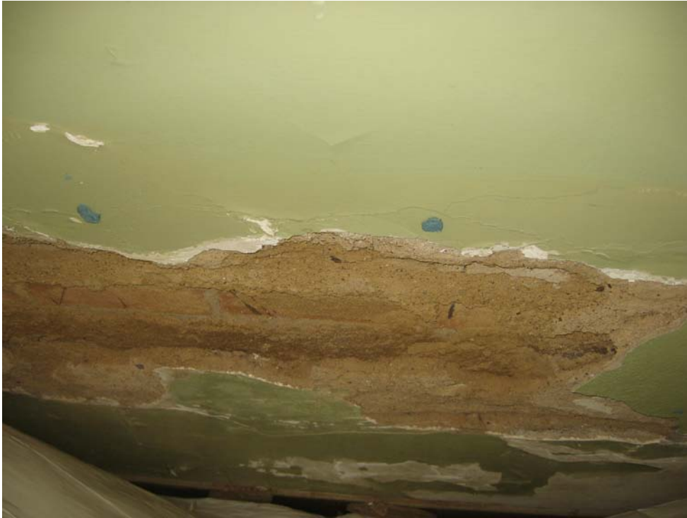
Photo P21-1 – Damaged plaster on inside face of west wall, west stair between First Floor and Basement.
