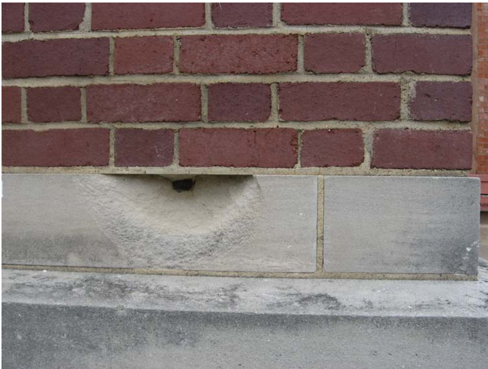
Photo P14-2 – Spalled piece of limestone with exposed anchor, southeast corner.
