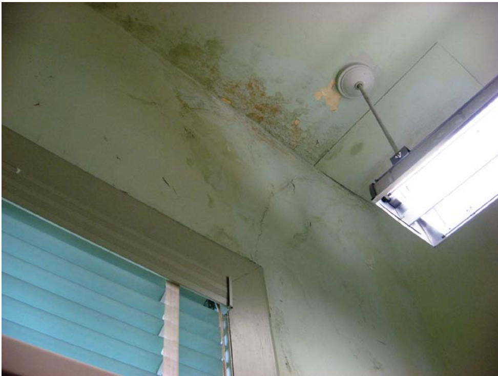
Photo P21-1 – Damaged plaster on inside face of west wall, west stair between First Floor and Basement.
