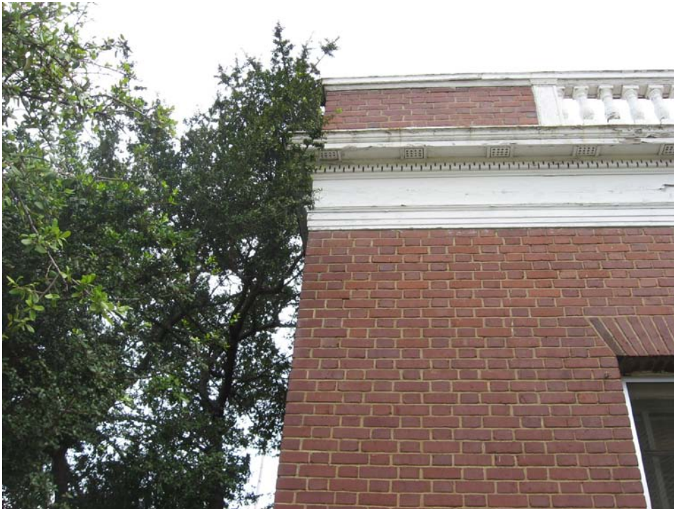
Photo P12-2 – Tree branches in contact with building, southwest corner.
