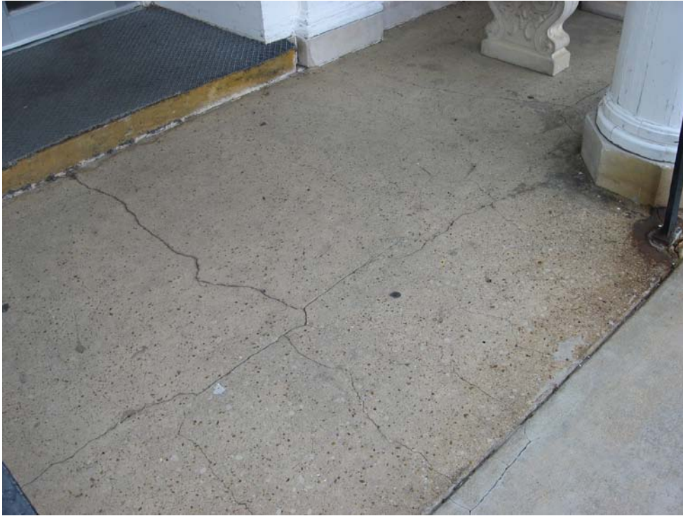
Photo P13-1 – Cracks in concrete at entry porch.
