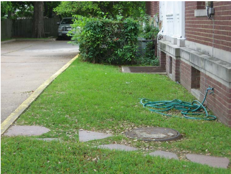
Photo P11-2 – Grade along North Elevation slopes back toward building.
