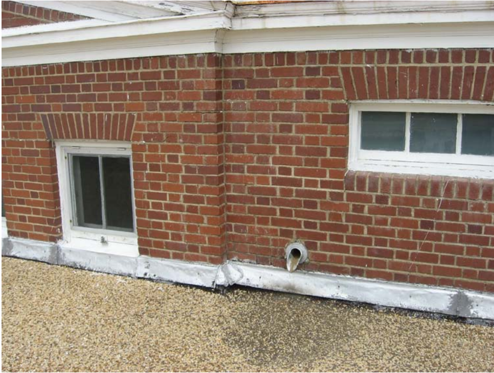
Photo P16-1 – Water from upper roof is deposited onto lower roof.
