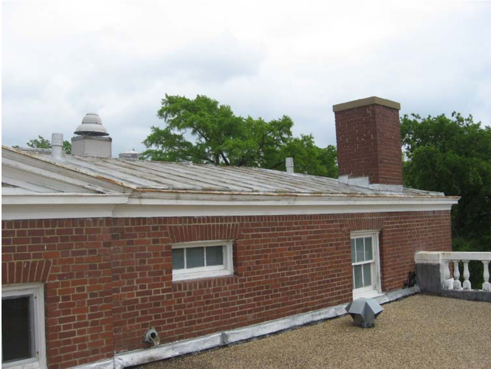
Photo P5-1 – Perimeter of upper roof is sloped, and transitions to flatter section over center portion.
