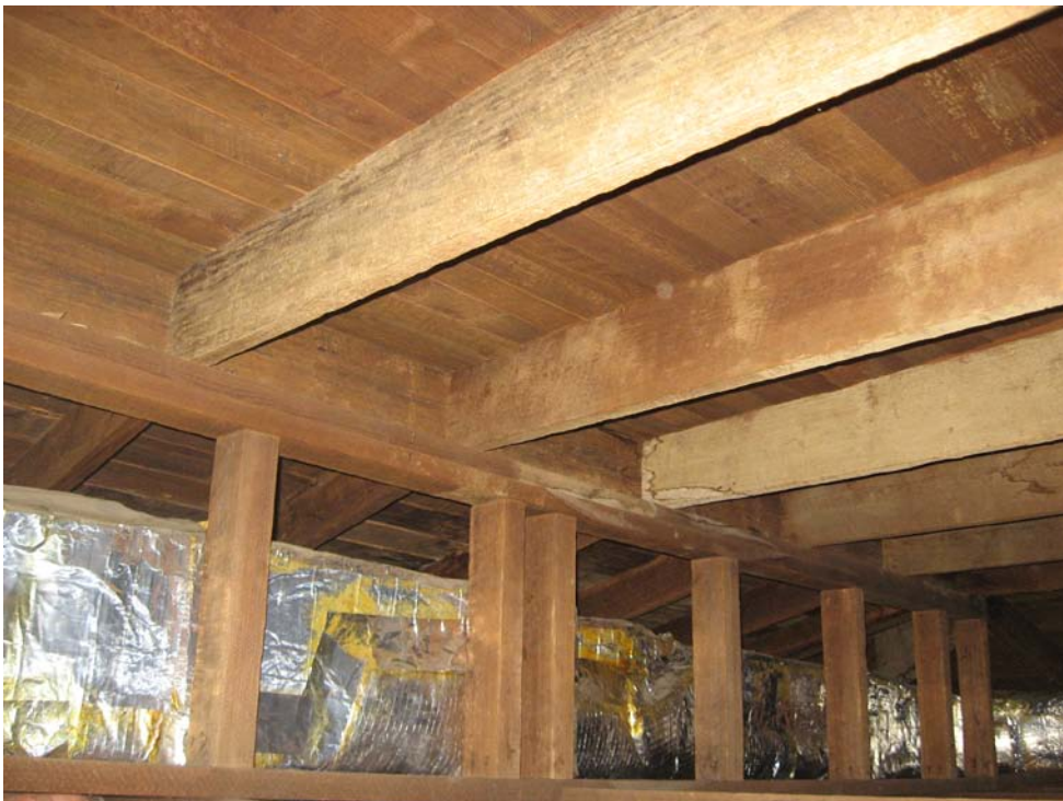
Photo P5-2 – 2x4 wood stud wall under transition at roof over Second Floor.
