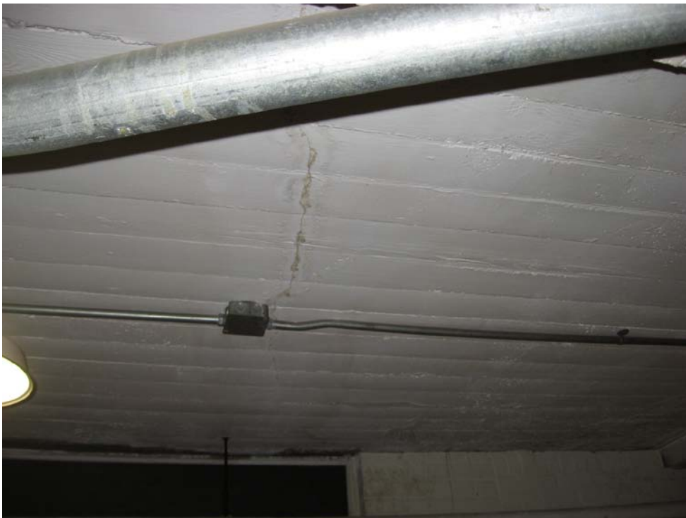
Photo P19-2 – Crack in underside of First Floor slab, east side of building.
