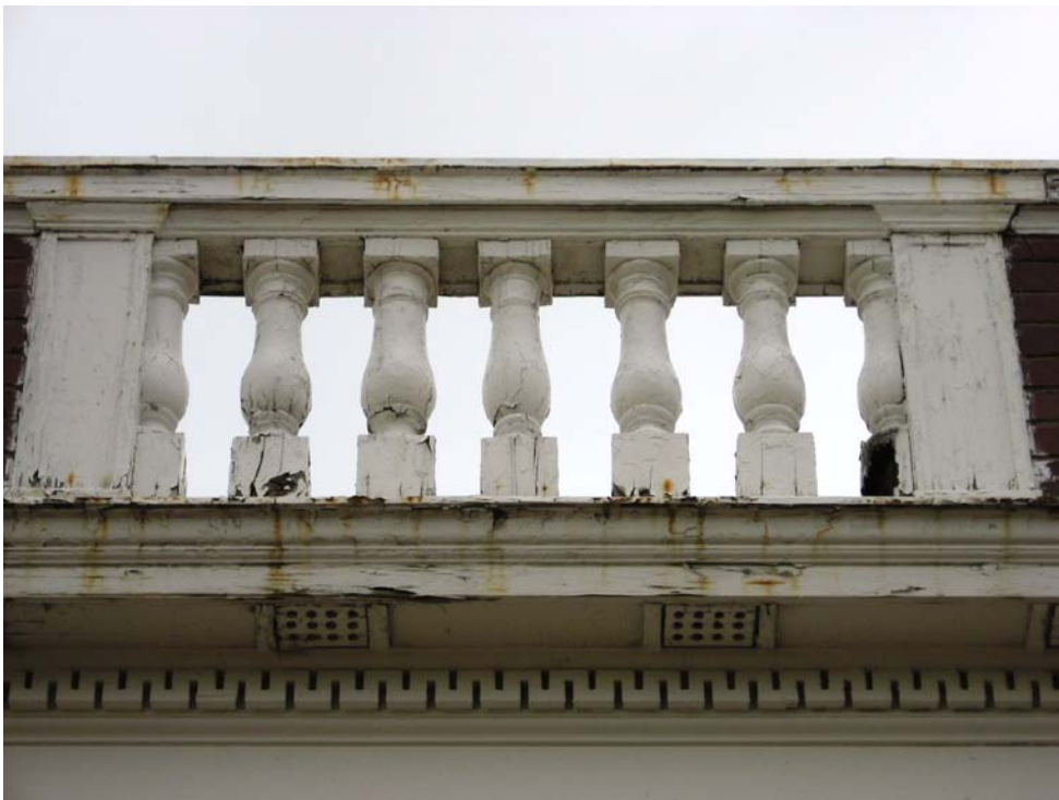
Photo P6-2 – Wood balustrades at parapet wall around low roof.
