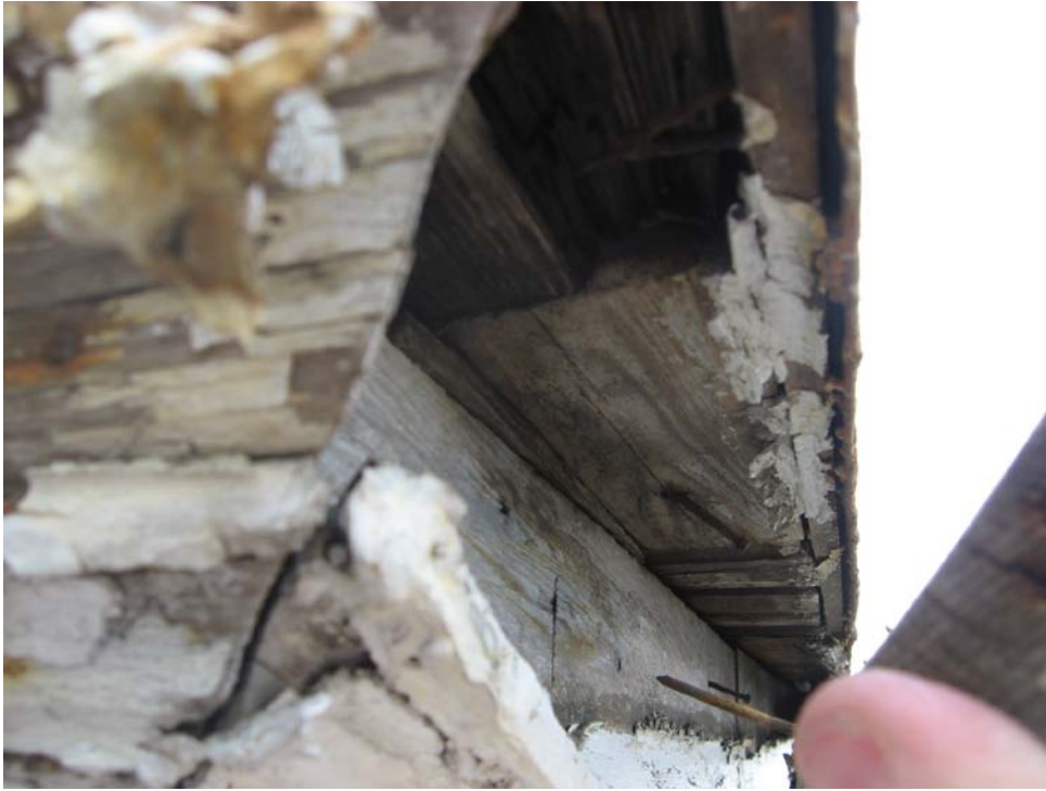
Photo P18-1 – Loose section of wood trim along upper roof, North Elevation.
