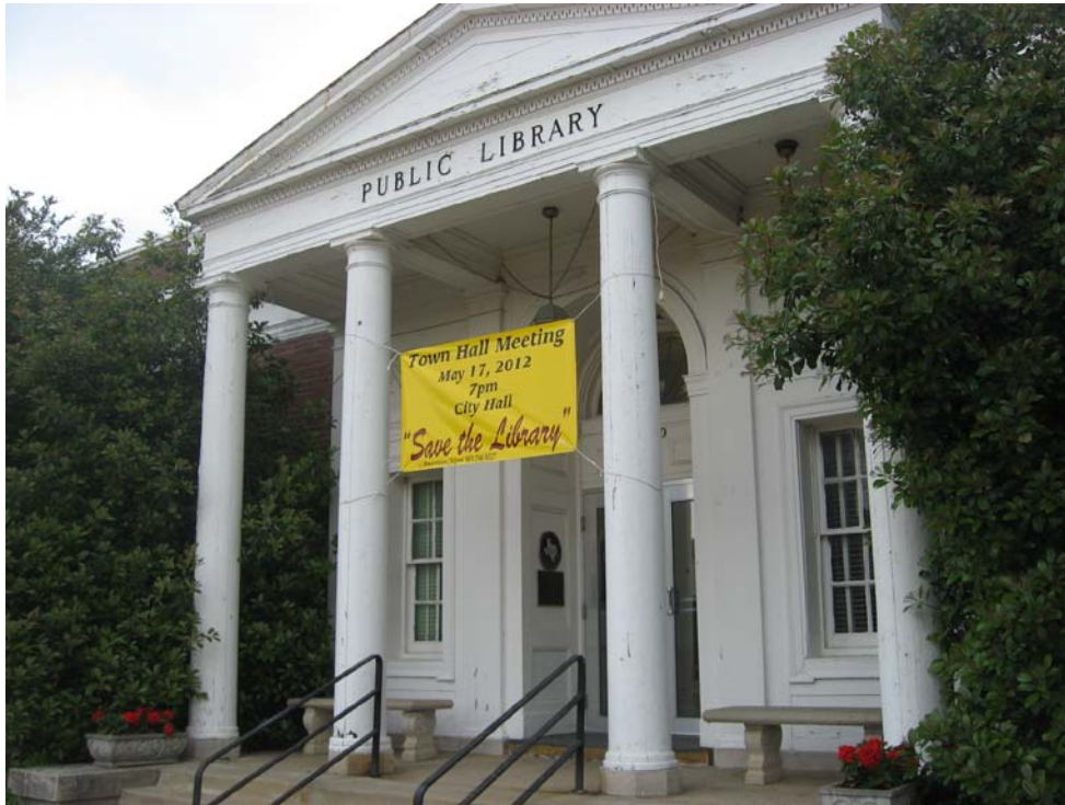
Photo P7-1 – Wooden Doric-style columns at entry portico, West Elevation.
