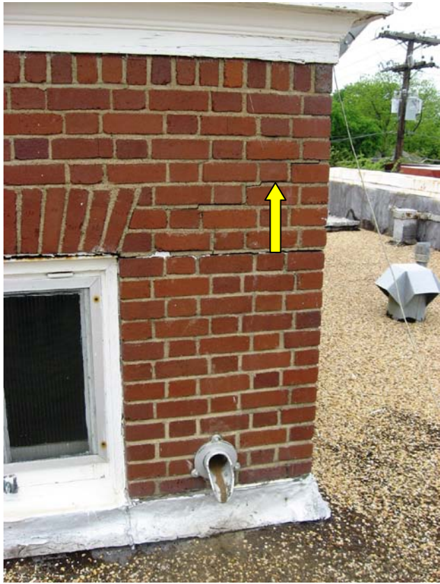
Photo P10-1 – Stair-stepped cracks at northwest corner.
