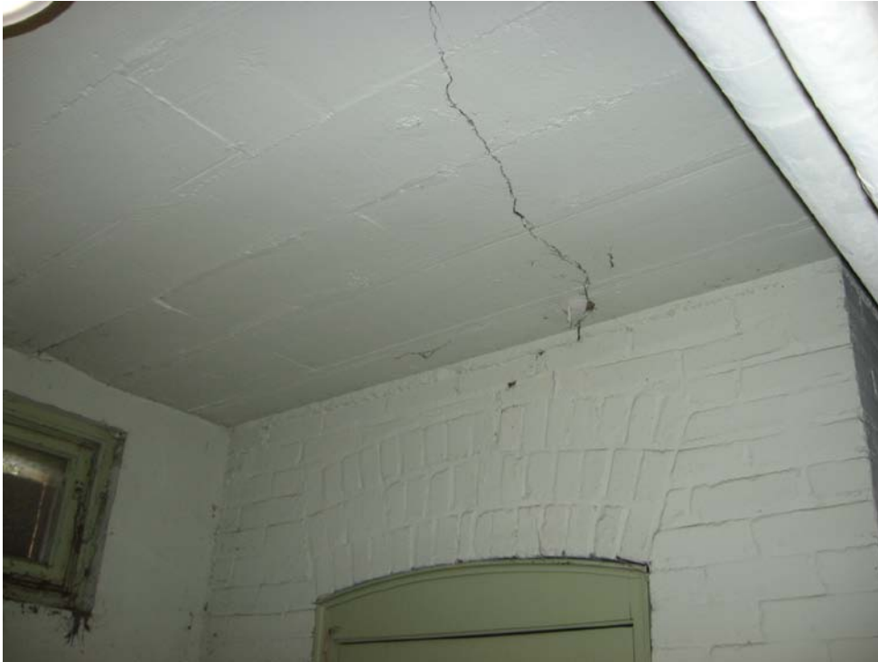
Photo P19-1 – Crack in underside of First Floor slab, northwest corner.
