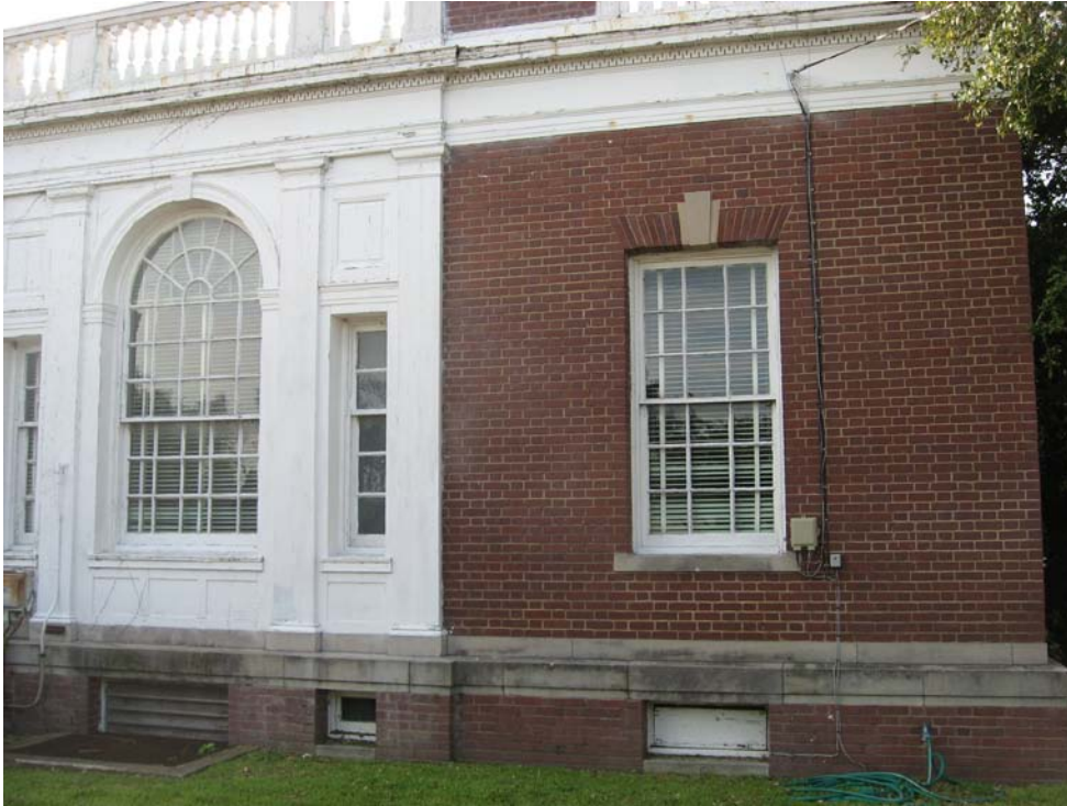
Photo P2-1 – Masonry window openings with limestone keystone and sill, and jack arch lintel.
