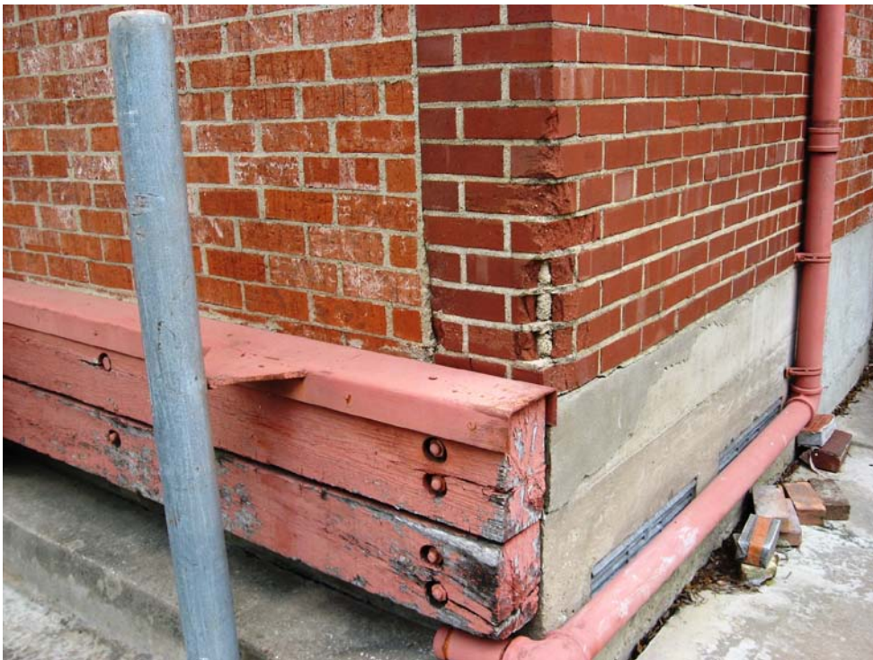
Photo P15-2 – Broken brick at northeast corner of east addition.
