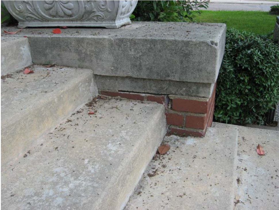
Photo P14-1 – Deteriorated brick mortar joints, south abutment at entry steps.
