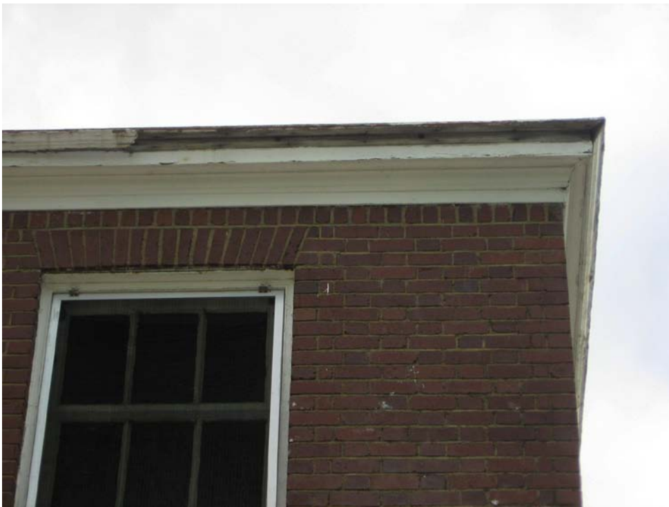
Photo P18-2 – Missing section of wood trim, upper roof, East Elevation.
