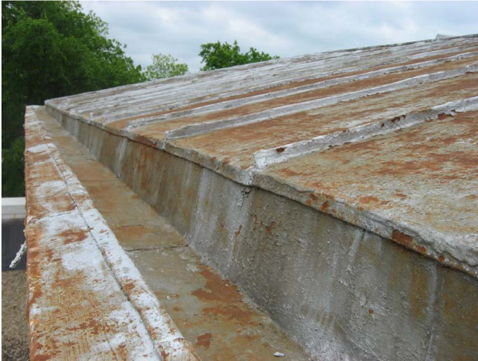
Photo P6-1 – Concealed tin-lined gutter at upper roof. Note deteriorated coating and corrosion on tin.
