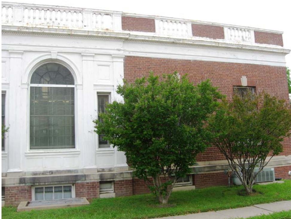
Photo P7-2 – Eastern portion of South Elevation. Note wood-trimmed elements.
