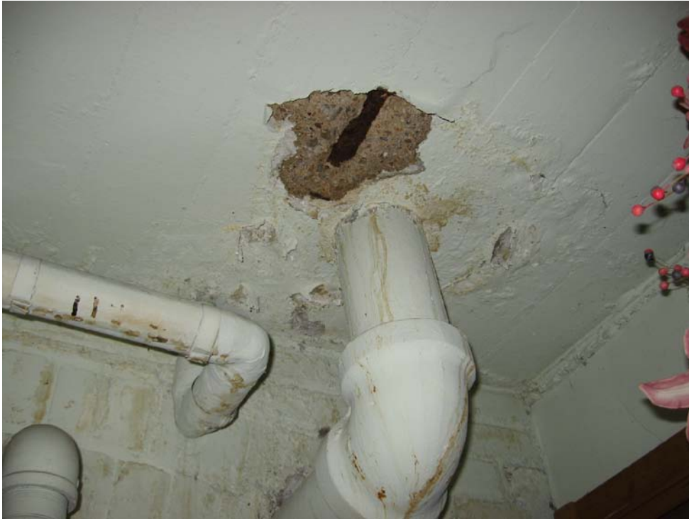
Photo P20-1 – Exposed and mildly corroded reinforcing steel at underside of First Floor slab.
