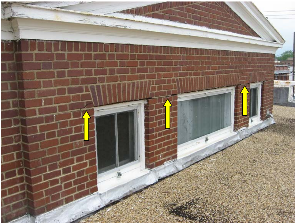
Photo P8-2 – Deteriorated mortar joints and broken brick units, North Elevation, Second Floor.
