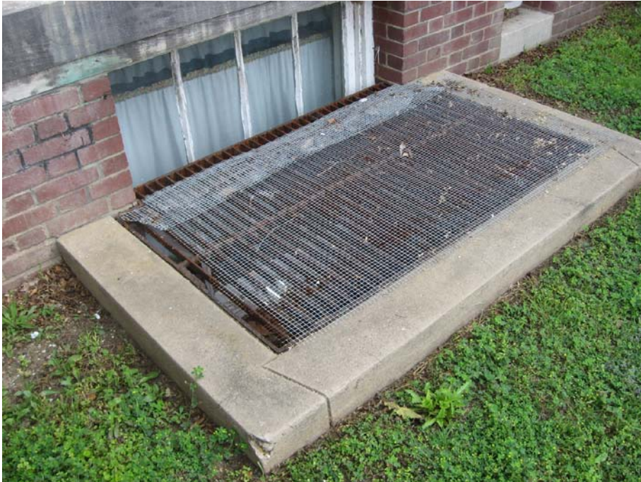
Photo P3-1 – Areaway at South Elevation.
