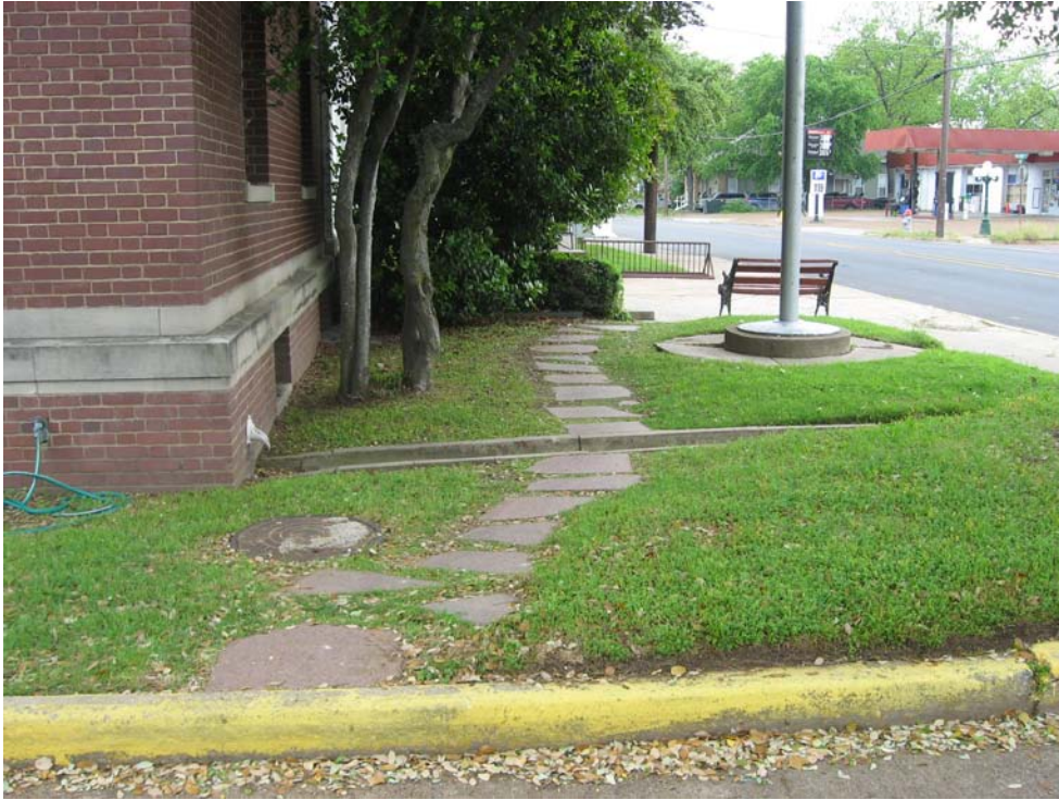
P12-1 – Grade and concrete drainage channel slope back toward building, West Elevation.
