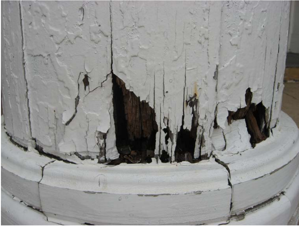
Photo P11-1 – Deteriorated wood at column surround, entry portico, West Elevation.
