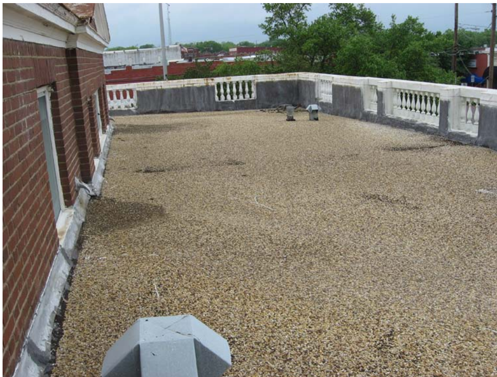
Photo P4-2 – Lower portions of the roof slope toward the north and south exterior walls.
