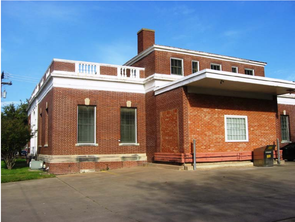
Photo P8-1 – Addition to east side of building. Note masonry infill at previous openings.
