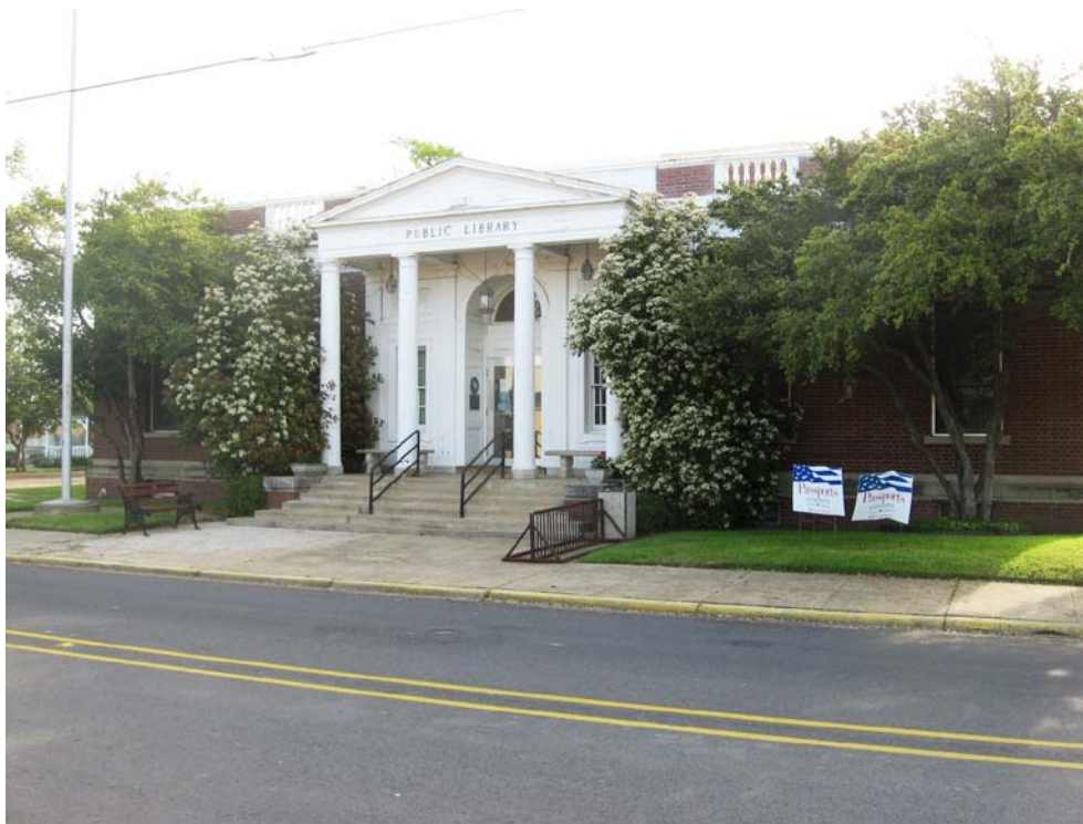
Photo P1-1 – West Elevation, Commerce Public Library.
