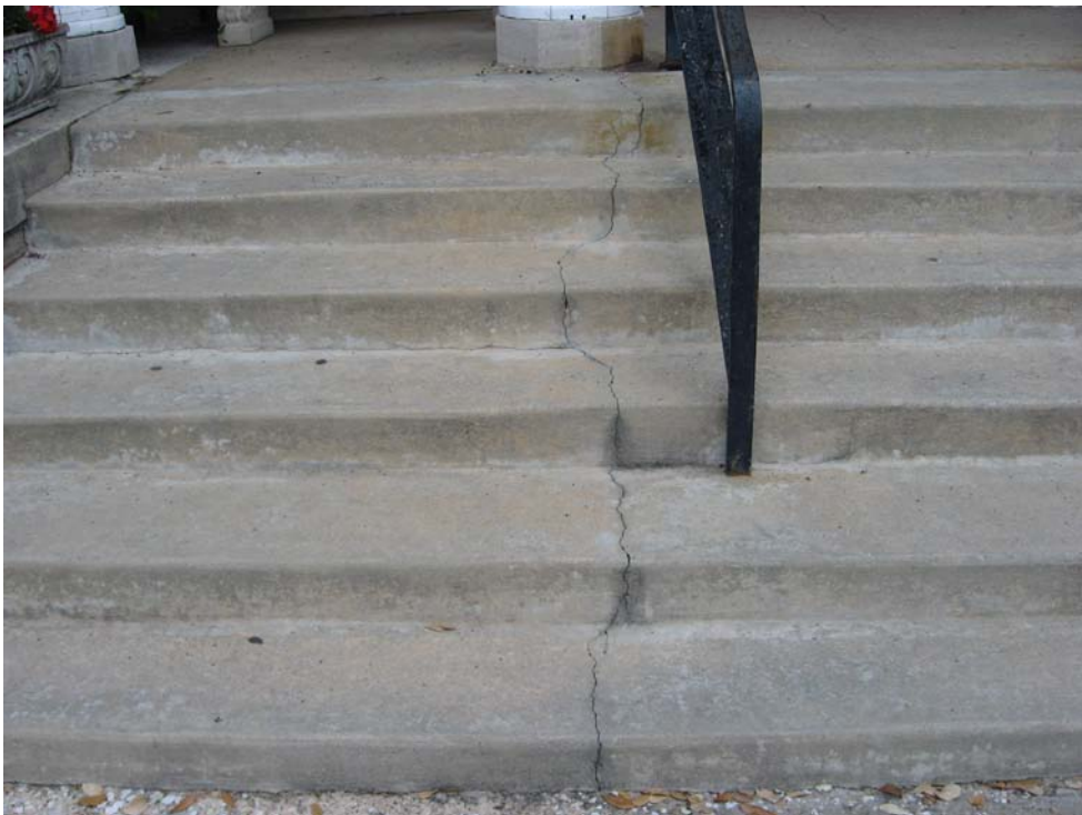
Photo P13-2 – Cracks in concrete entry steps.
