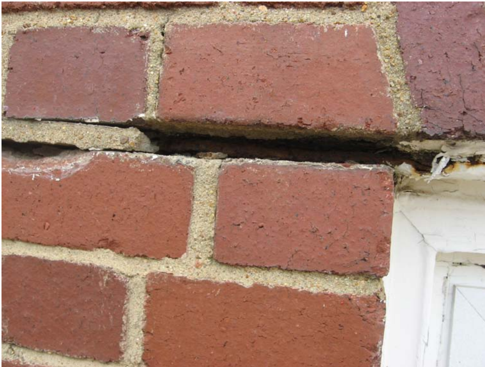
Photo P9-2 – Corrosion on embedded steel lintel.
