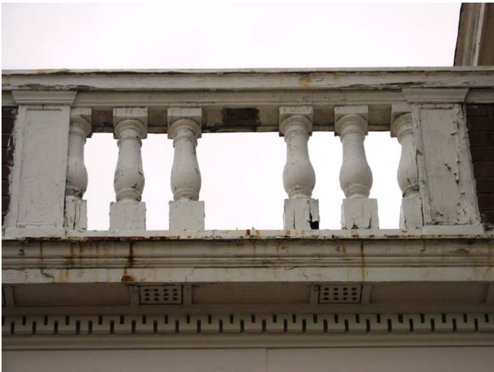
Photo P17-2 – Missing baluster.
